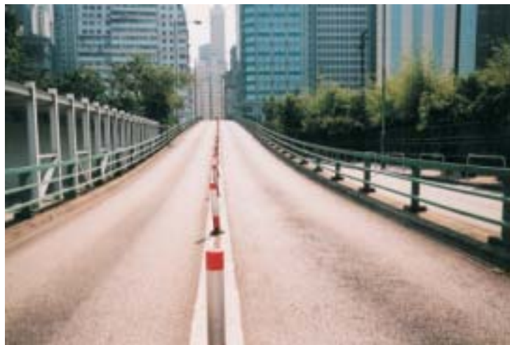
Figure 9.2 – First generation P1 three-rail steel parapet
