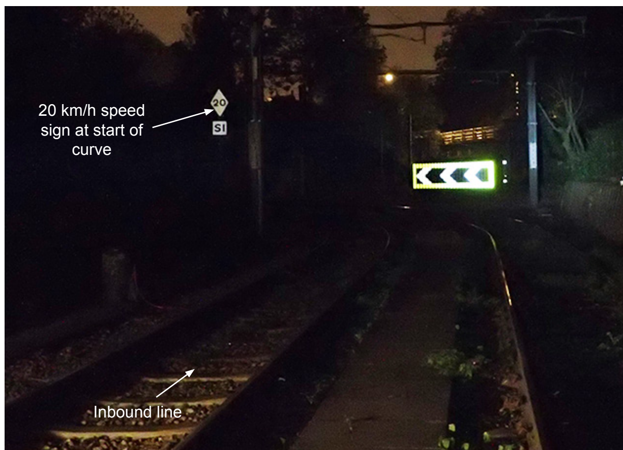
Figure 54: Chevron sign fitted as part of the signage changes at Sandilands south curve after the accident
